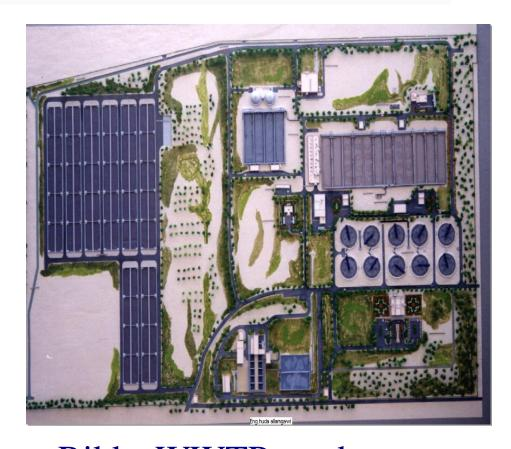
Rikka WWTP produce treated water of 280,000m3/day by using sand filters.
