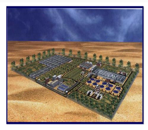
• Kabbed WWTP have a capacity of 180,000 m3/day it will be expanded to 270,000 m3/d it produce a tertiary treated water of 175,000 m3/day by using disc filters.
