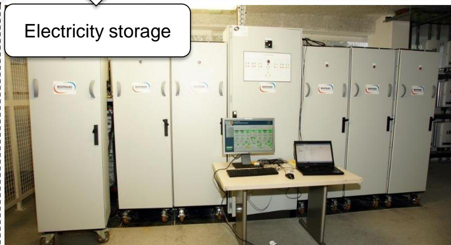
6 Kangoo batteries ZE – 66 kW / 66 kWh
