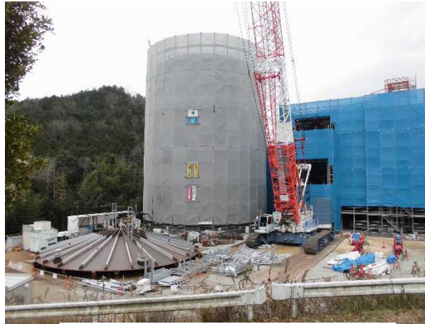
Methane fermentation tank installation status
