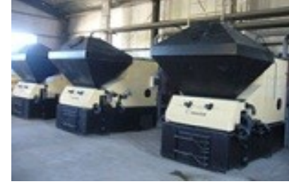
High-efficiency Heat only Boilers, Suuri-Keikaku, Mongolia
