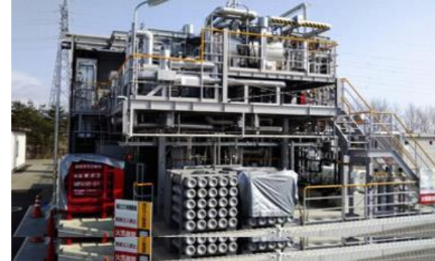
Pilot plant of a new NH 3 production process using renewable H 2 as raw material.
