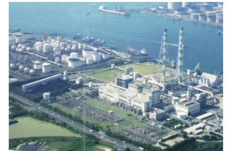
Mizushima power plant NO.2 Unit (156MW)
